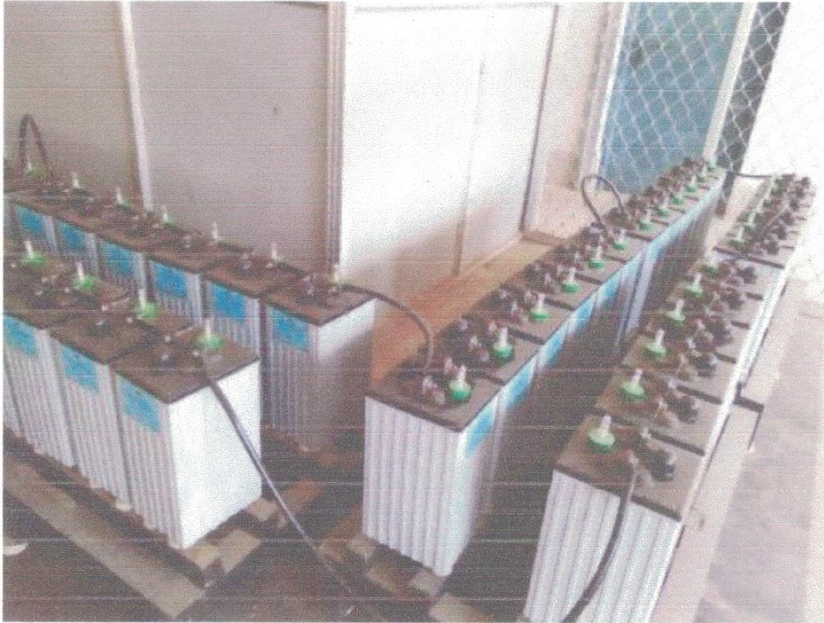
Figure shows battery installed for uninterrupted power supply.
